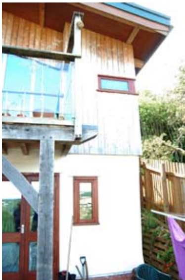
Fig. 5.34: Jim Carfrae's home is a combination of conventional lime render and untreated FSC Western Red Cedar cladding.
