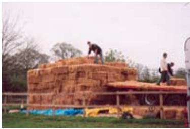
Fig. 5.31: Straw bales being delivered to Paul Douglas's site.
