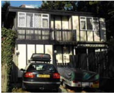
Fig. 2.22: A typical Segal method house at Lewisham.
