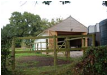
Figs. 4.22 and 4.23: Before the build, the concrete slab with rammed tyre foundations and horsebox. And after, the finished garage looks at home in the farmyard.
