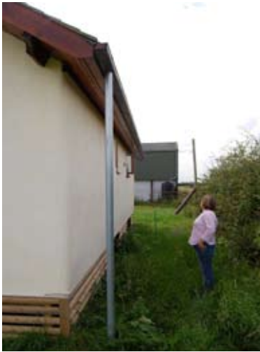
Fig. 4.51: Carol Atkinson inspects the lime render and wooden guttering on her straw bale caravan.
