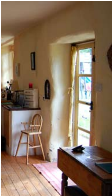
Fig. 5.11: Ten per cent of the footprint of The Straw House is taken up by its thick walls.
