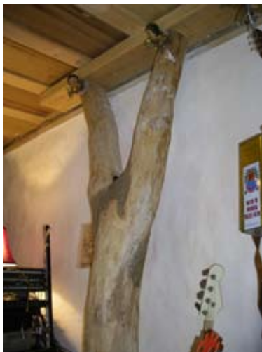
Fig. 4.62: One of the Strawdio's load bearing tree trunks.
