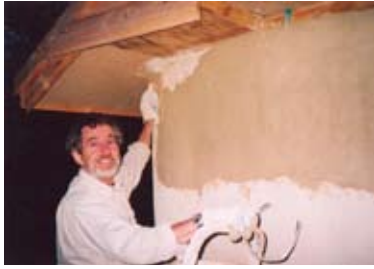
Fig. 4.21: Paul Douglas applying lime render to his straw bale garage.
