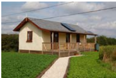
Fig. 4.52: The straw bale cabin with its large south facing verandah.
