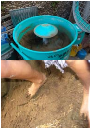
Figs. 5.32 and 5.33: Rik's render mixer (top) couldn't reproduce the mixing power of stamping volunteers.
